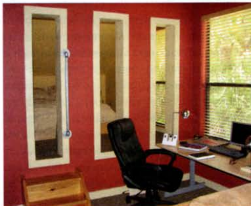
TUCK ME IN: A sleeping "nest" off the home office in Ed Binkley's own Florida residence makes clever use of what would otherwise be an unused cavity in the framing.
